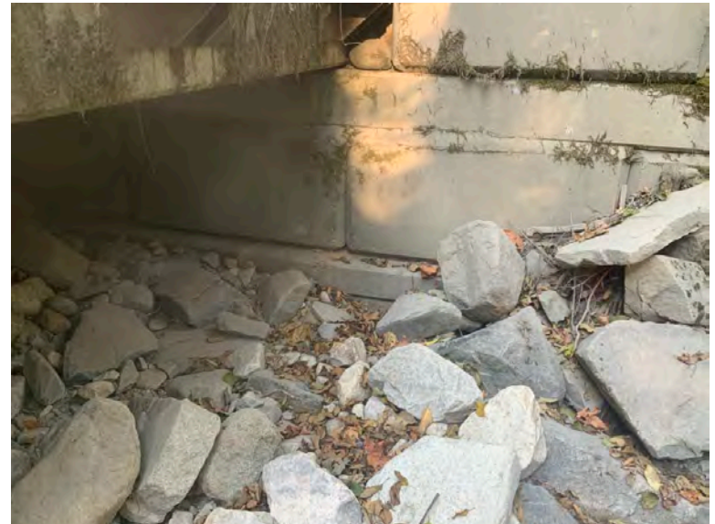
Left Bank Abutment when facing downstream
