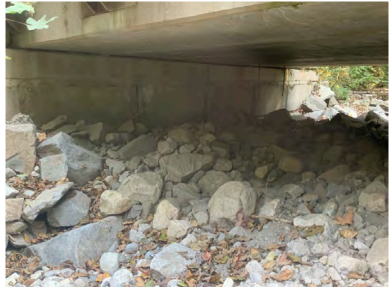
Left Bank Abutment when facing downstream
