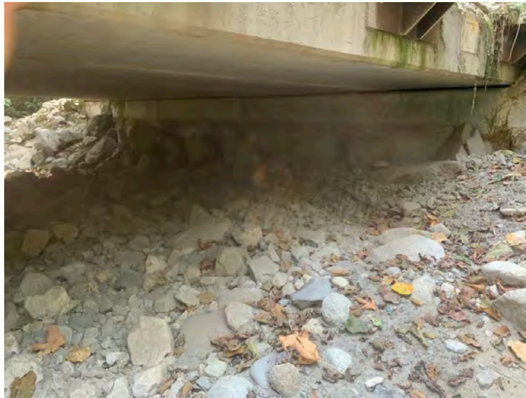
Right Bank Abutment when facing downstream
