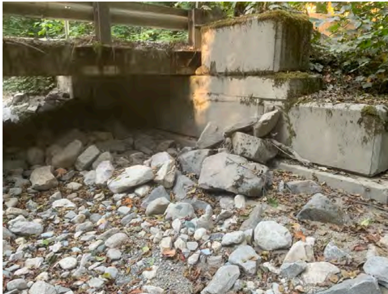
Left Bank Abutment when facing downstream
